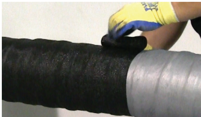
For some exposed applications, or applications requiring additional mechanical protection, Trenton recommends the use of an outerwrap. Trenton MCO™ moisture-cured outerwrap (shown above) provides excellent mechanical strength and quick curing times.
