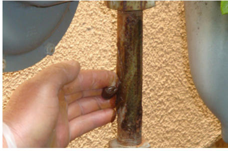
5. Pay special attention to applying primer in and around all angles and threads.
