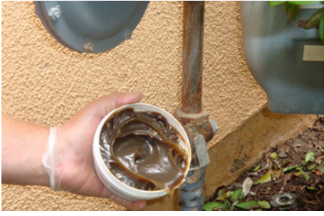
4. Hand apply the primer. Firmly rub and press the primer onto the surface to displace the moisture and ensure that the primer is adhering to the metal surface.
