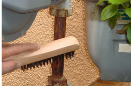
2. Wire brush so that the surface is free from loose rust, dirt and old, loose coating.
