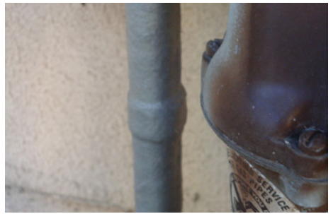
9. Inspect your work. Make sure all desired areas to be coated are completely covered. Remove and re-apply if needed.
