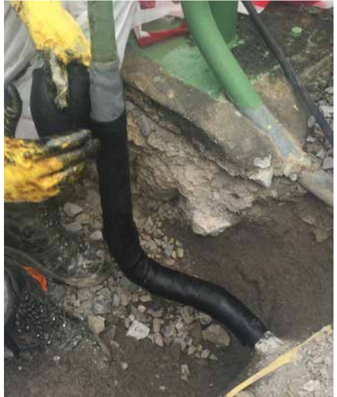
For irregularly shaped pipe or fittings, MCO 110 outerwrap has good conformability. The transition here shows how MCO 110 wrapped over Wax-Tape® #2 anticorrosion wrap will provide excellent protection against frost heave and possible mechanical damage.
