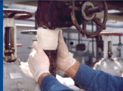
The STOP IT® Pipe Repair System includes a strong knitted fiberglass tape coated with fast setting urethane resins that are water activated. The system also includes FIX STIX™, a steel filled hand moldable epoxy that sets rock hard in only 20 minutes.
