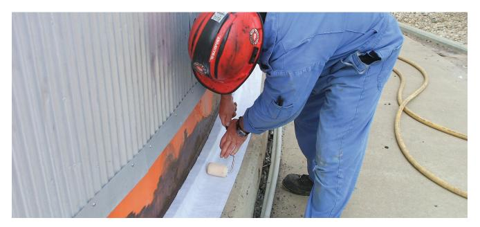
VISCOTAQ<sup>®</sup> EZ-WRAP can be used in environments and on substrates with an ambient or surface temperature up to +71° C/+160°. The product can be applied without significant surface preparation.
