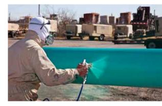
3M<sup>™</sup> Scotchkote<sup>™</sup> Abrasion Resistant Epoxy Coating (AREC) 328 is a proprietary new technology for the protection of steel pipelines from corrosion. Combining a traditional liquid epoxy with enhanced abrasion resistance, flexibility, and impact resistance, an AREC coating can be used in place of a conventional Abrasion Resistant Overcoat (ARO) or as a primary corrosion protection coating.
